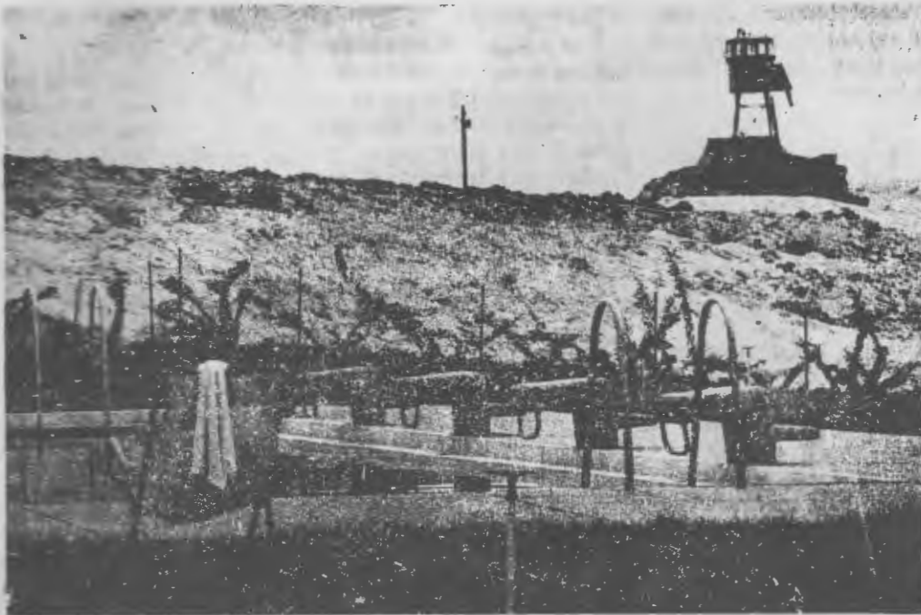
Swimming pool at a settlement in the Jordan Valley.
