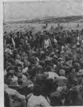
The dyke built
