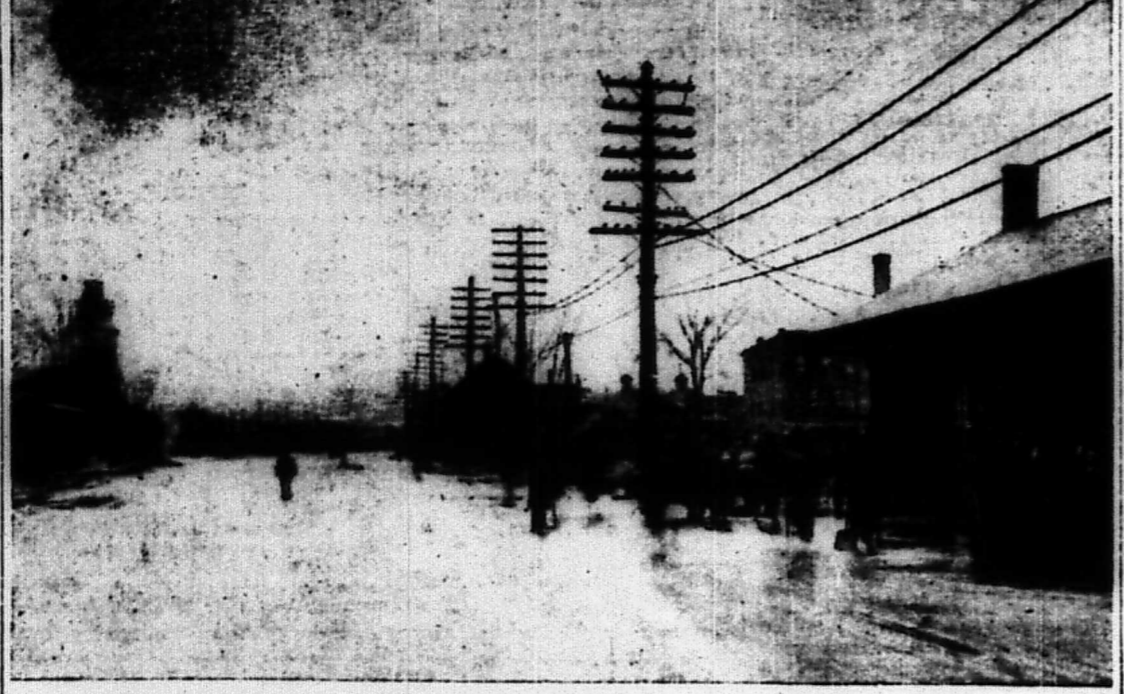
Looking Eastward Along the Inundated Tracks at the New York Central Station at Heckimer.
