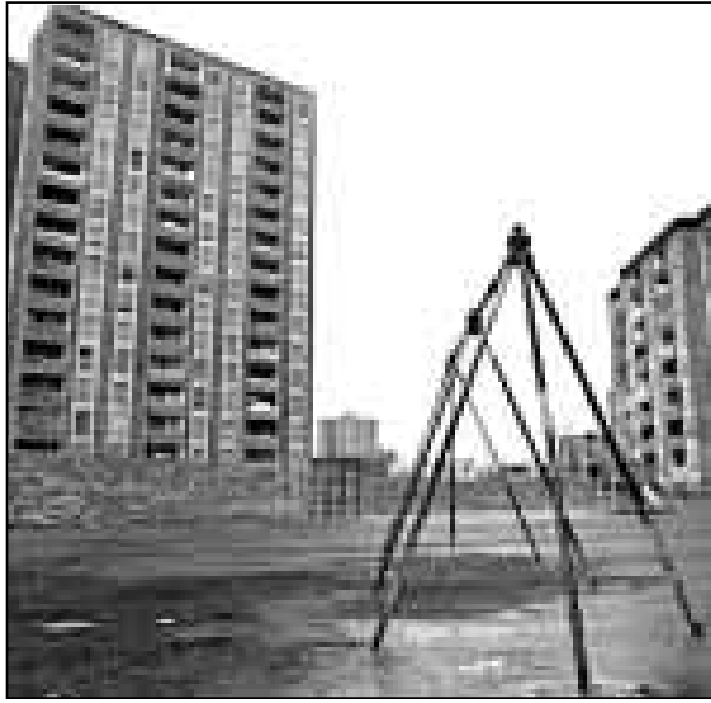
Demolition of towers could contaminate area with asbestos fibres
