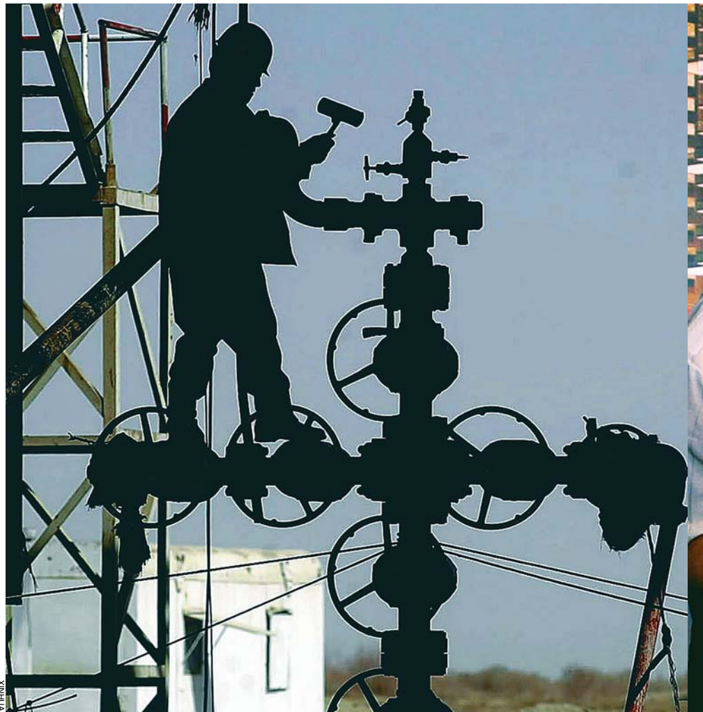
Construction of the west-to-east natural gas pipeline is underway
