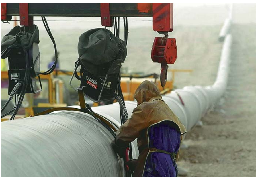
A west-to-east natural gas pipelining project is constructed to ease energy shortages
