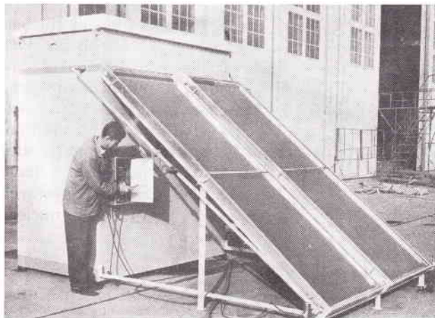
A solar bathhouse which can shower 20 people daily.
