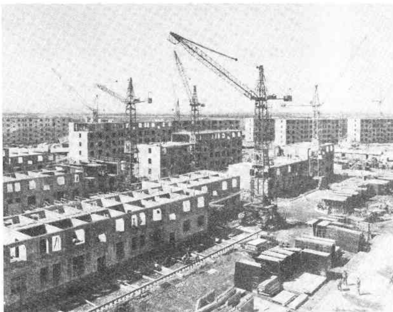
A new residential quarter under construction.
