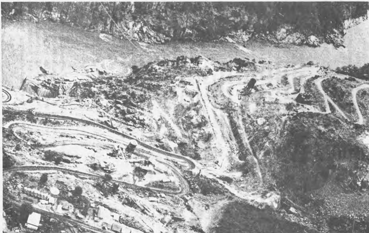
The Cabora Bassa dam site seen from the air. On the side of the cliff engineers have blasted out a hairpin bend road which is the only means of access to the site of the dam itself.
